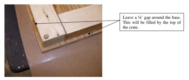
Once all four edge pieces are in place, rip two pieces of 2"x6" down to 2"x4" by 11" long. These will be attached to the base with four 2-1/2" decking screws in the locations shown in the next photograph.
