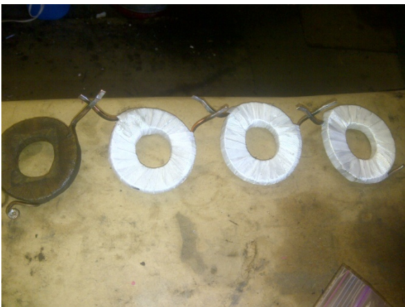
Three coils with new outer insulation
